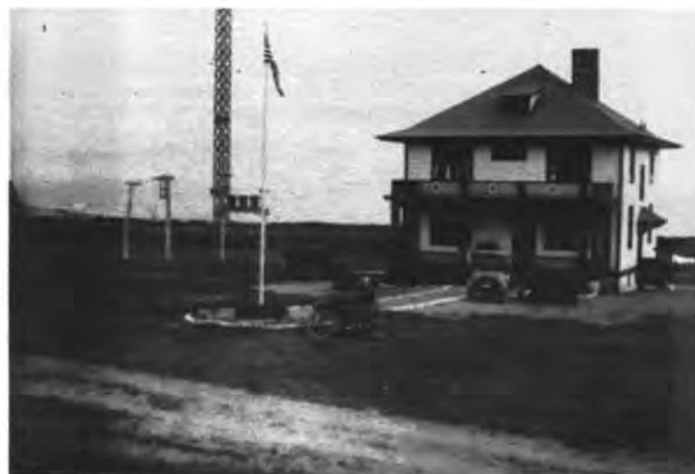
Seawall Remote Transmitter Site. Accirdubg ti "Hank" Grindle, that intrepid motorbike rider is the foreground is none other than Carl Herr !. Photo - [Fred Grindle ]
